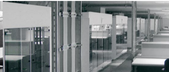
Cool-Rack connected to four-way units
